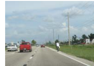
Example of the lack of multi-modal options along US 41, Tamiami Trail
