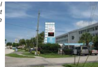
Fawcett Memorial Hospital in Port Charlotte
